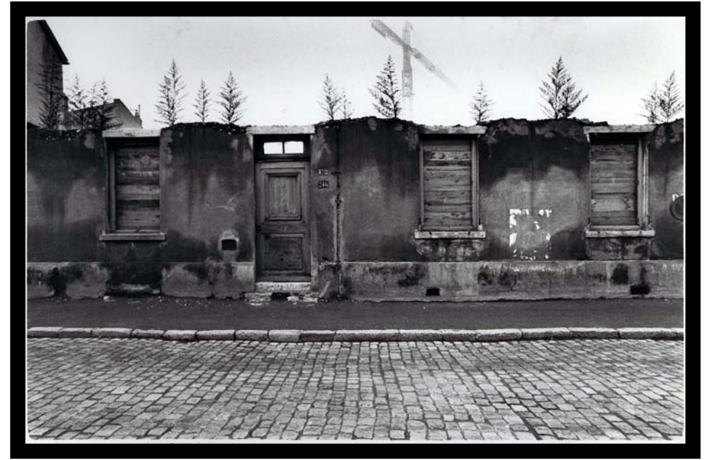
Lyon - chantier avenue Paul Santy, 1972
