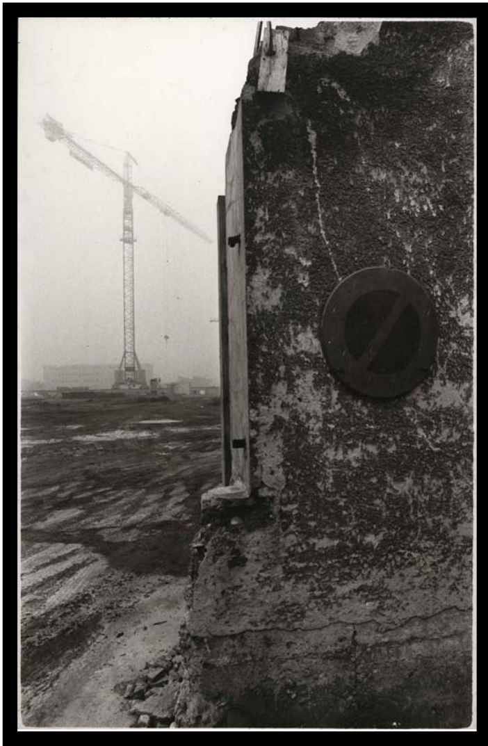
Lyon - chantier avenue Paul Santy, 1972
